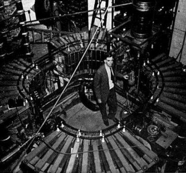
„Race track” synchrotron by D. Crane (Univ. of Michigan, 1949)
